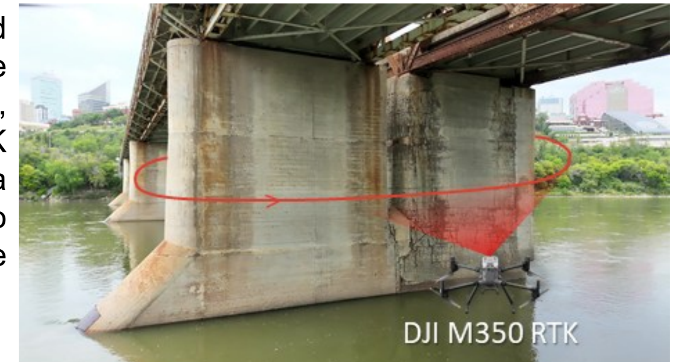
Figure 4: Field data collection on the pier.
