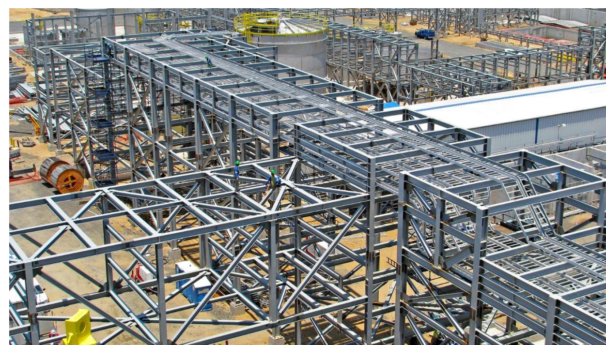
Figure 1: Typical pipe rack structures in industrial facilities supporting pipelines and transferring loads to foundation systems Sources: Sunway Steel (sunwaysteel.com); VisSteel (vissteel.com.vn)
